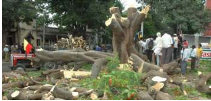
Plate 9. Loading Log from Avenue Trees for Road Widening
